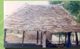
Construction of the new thatched dairy shed
