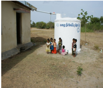
A School Rain Water Harvesting Tank
